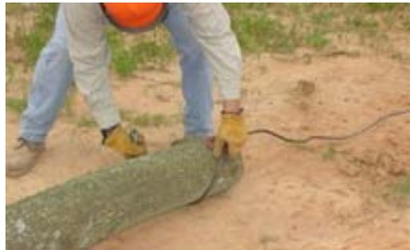
5. Secure the winch rope through the loop never on the rope itself.
